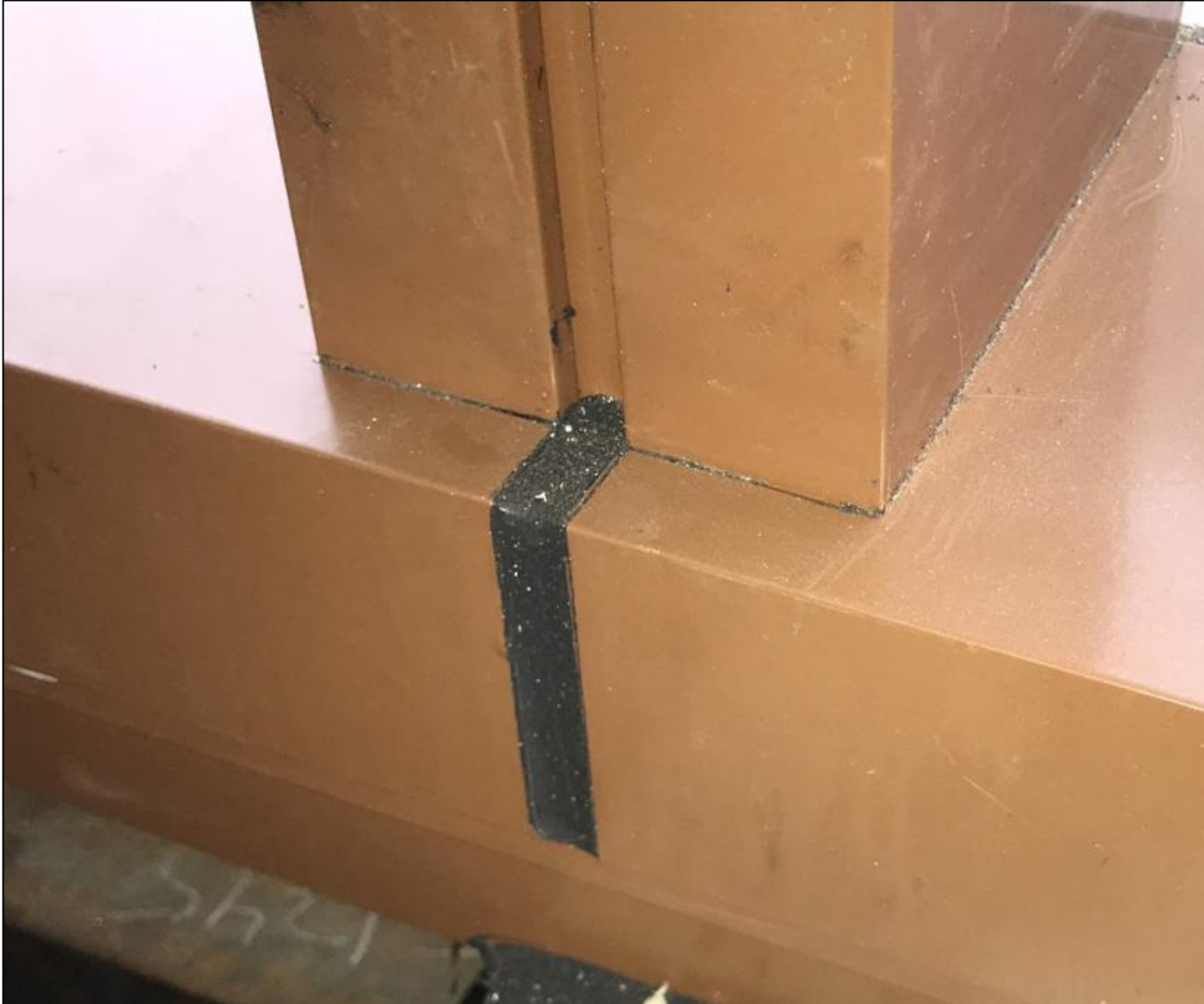
Sealing the bottom joints with Schuco Flex
