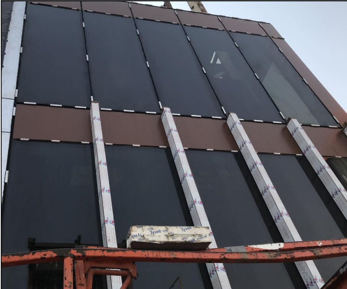
Installing all panels
