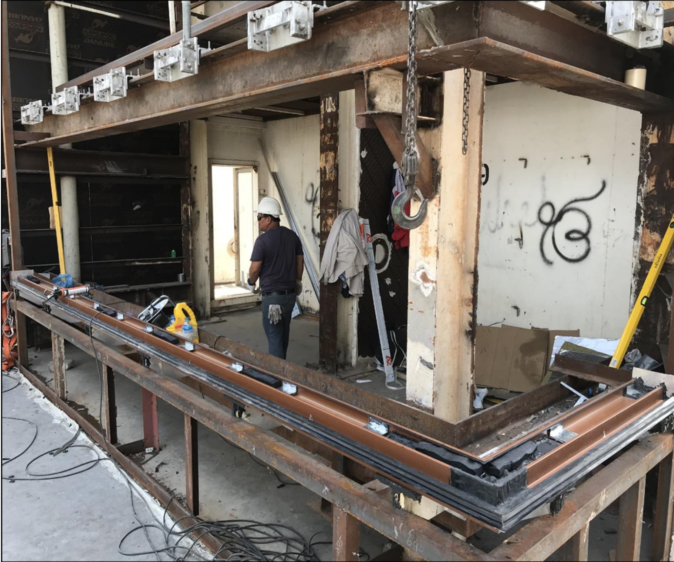
The installation of the starter gutter profile
