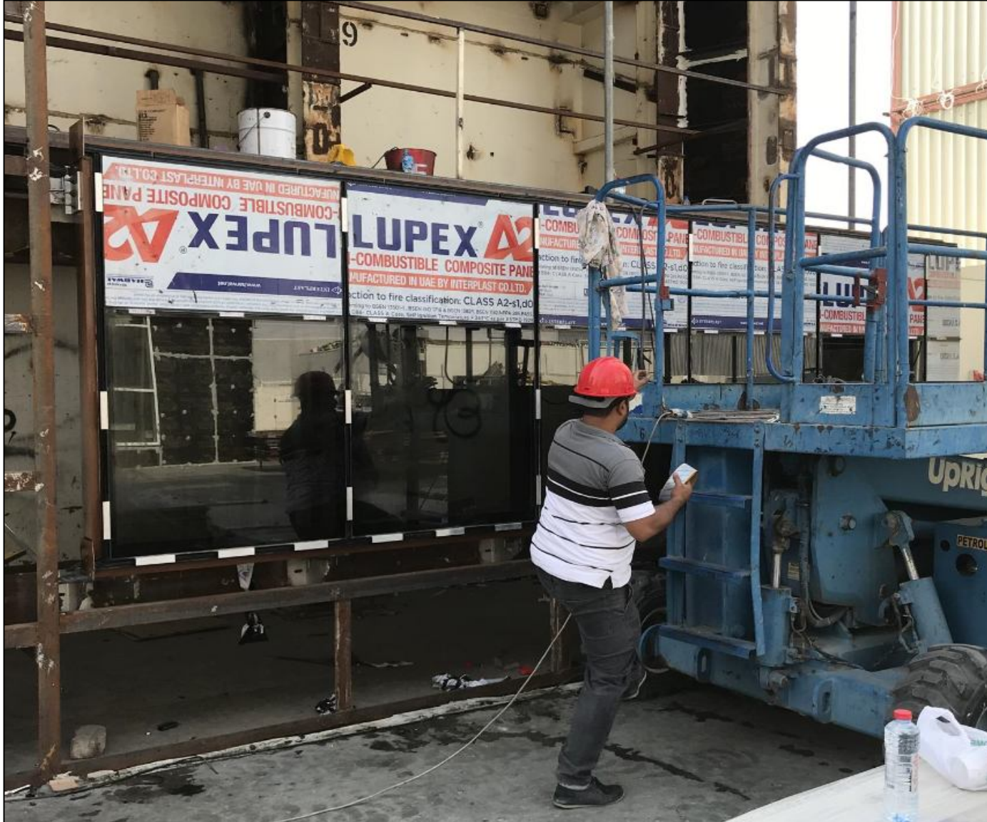
Installing and aligning the panels
