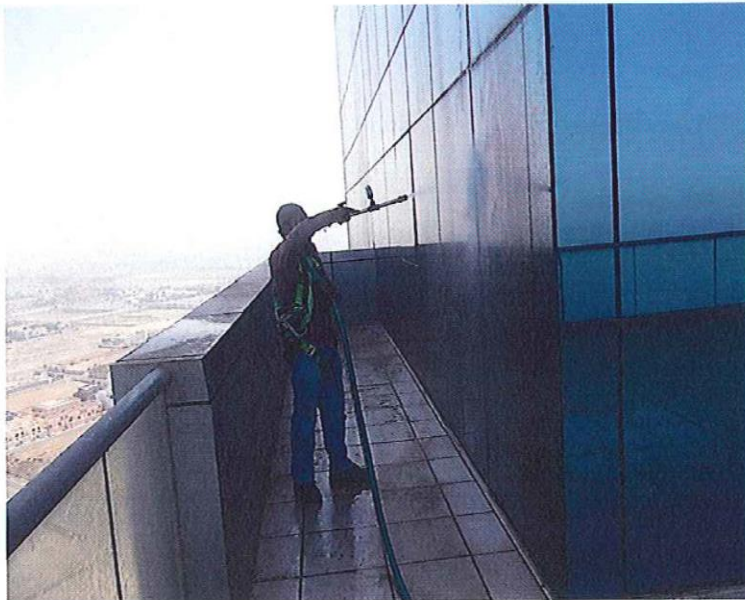
Photo 2 Testing on the balcony façade
