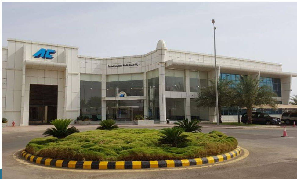
AACC Building - Jeddah
