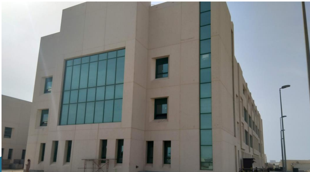
National Guard Housing - Dammam
