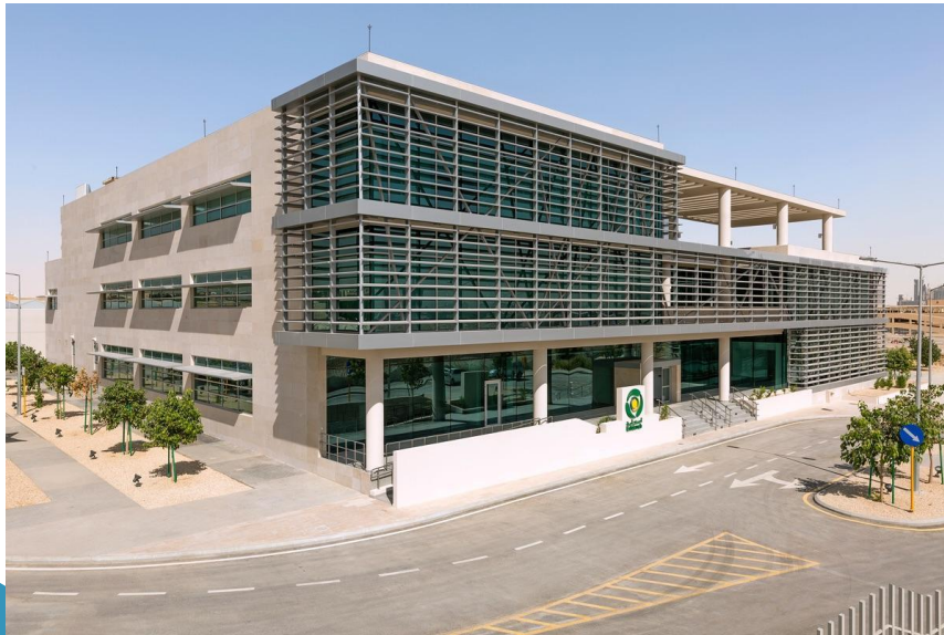
Sabic GreenHouse - Riyadh
