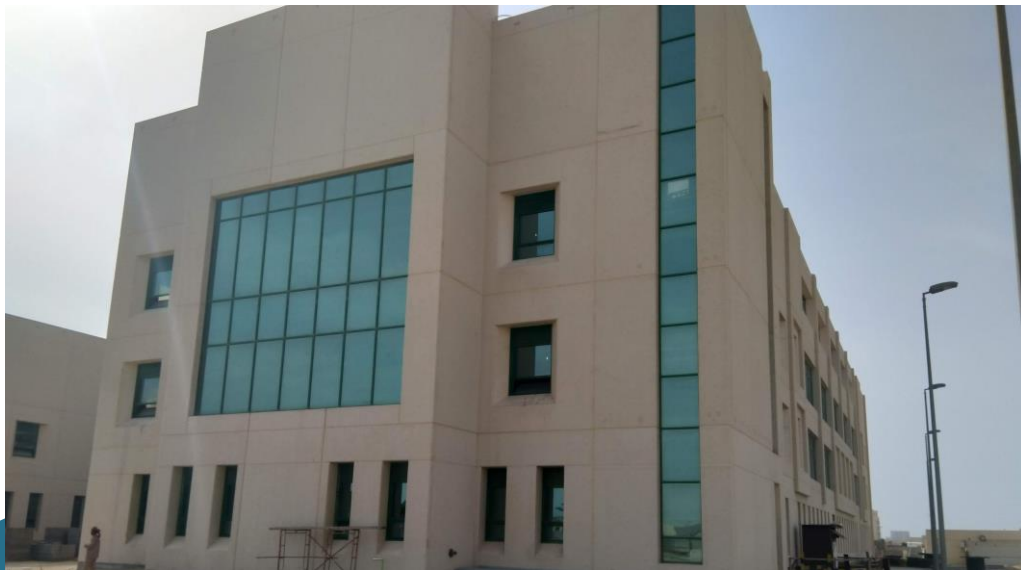
National Guard Housing - Dammam
