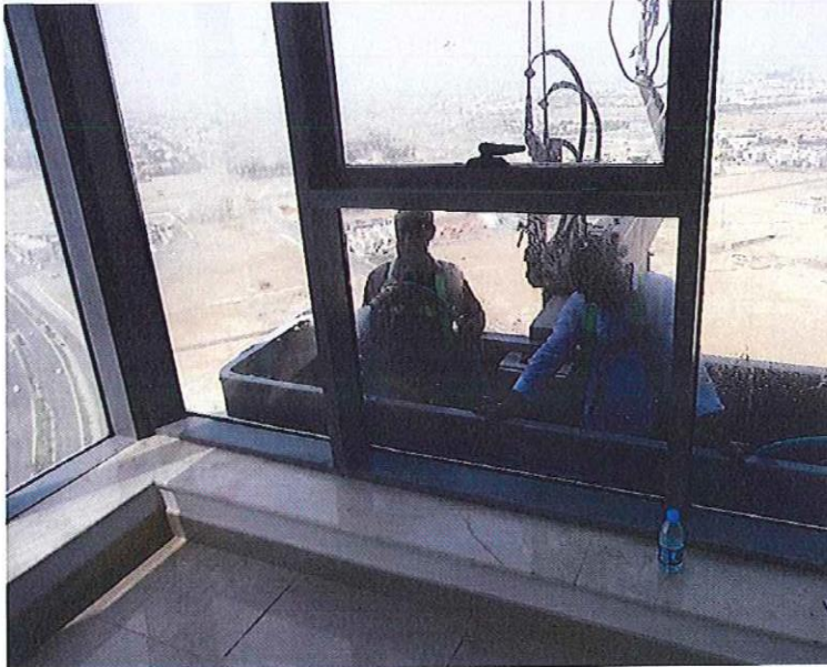
Photo 1 Water penetration test in progress
