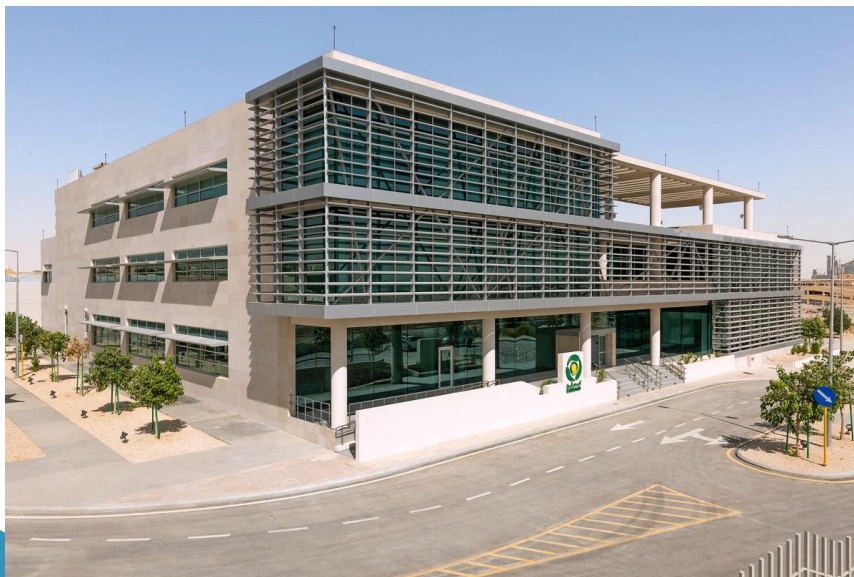
Sabic GreenHouse - Riyadh
