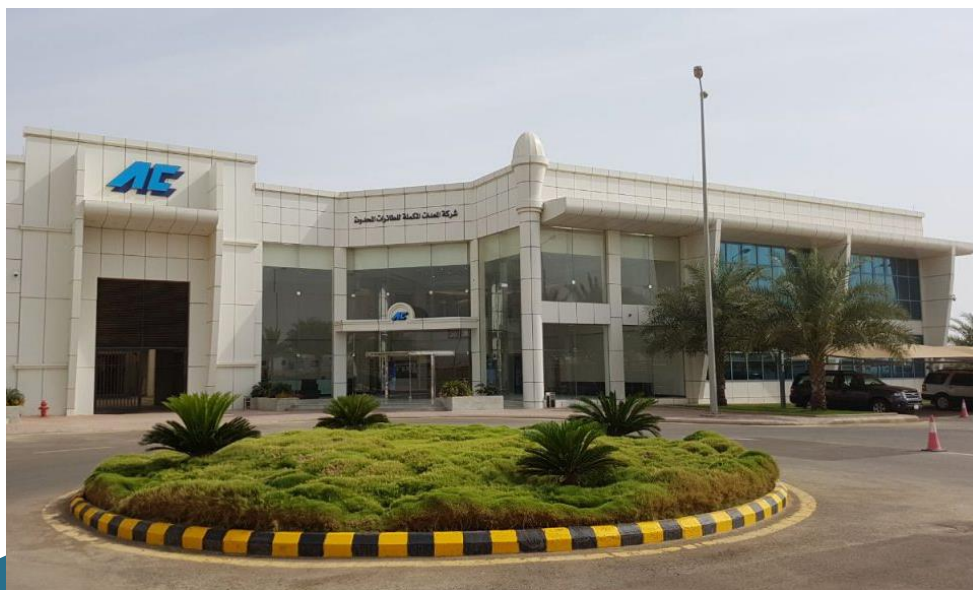
AACC Building - Jeddah
