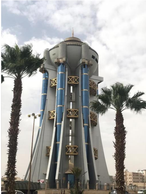
Water Tank Tower – Khamis Mushayt
