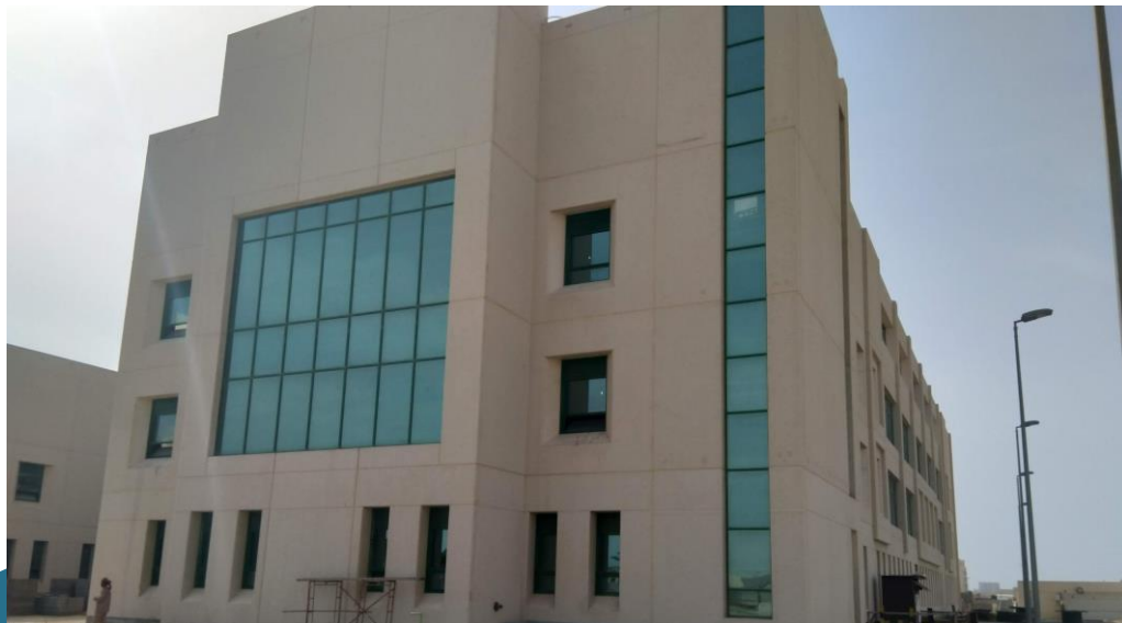
National Guard Housing - Dammam
