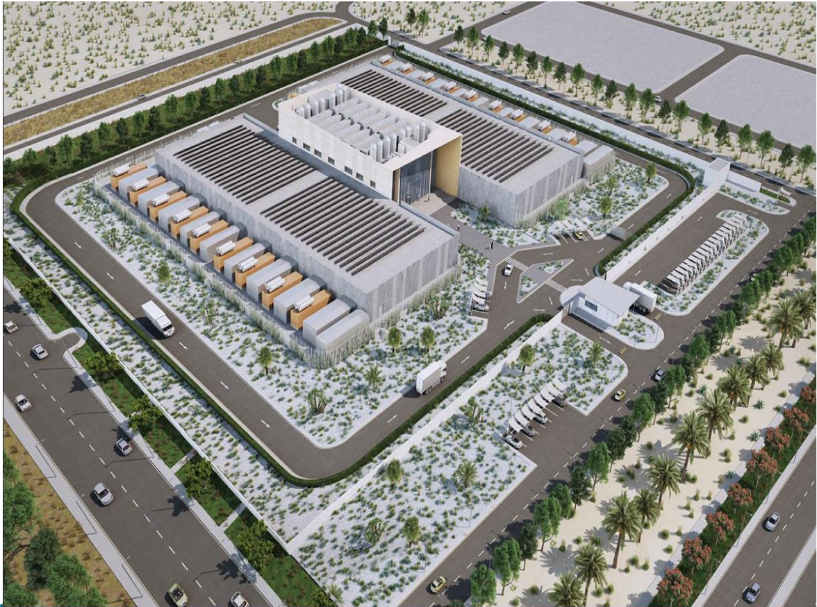
Sahayeb Data Centers (DC1, DC2, DC3) - Damman
