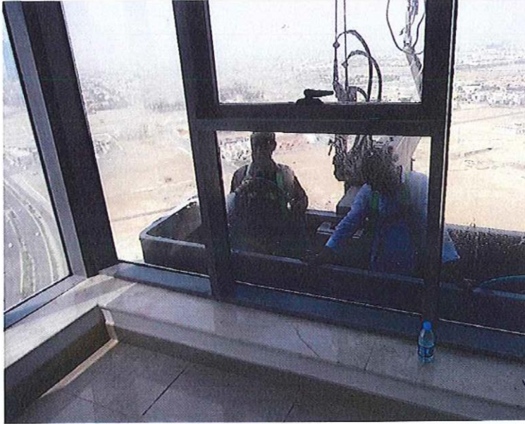
Photo 1 Water penetration test in progress
